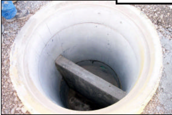
Sewage Inlet Structure Repair at Airport
