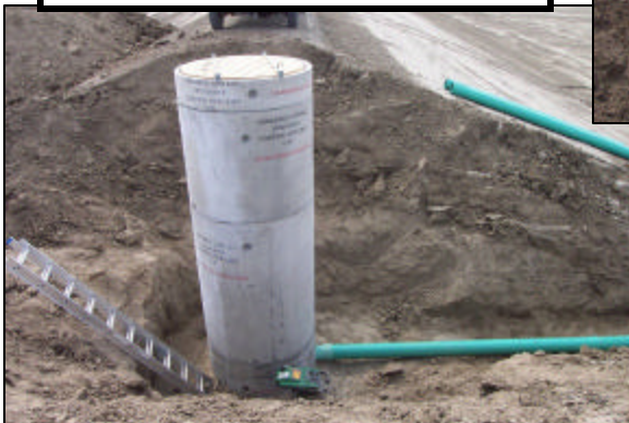
Monarch Sewage Project
