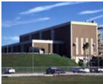
Solid Waste Facility
