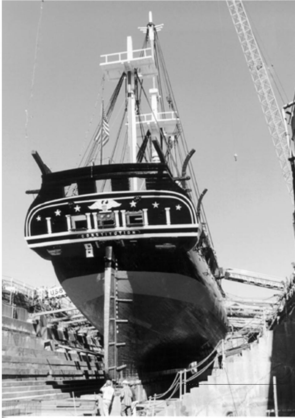
The Constitution's fine and fast sailing hull is ready for undocking, September 25, 1995.
